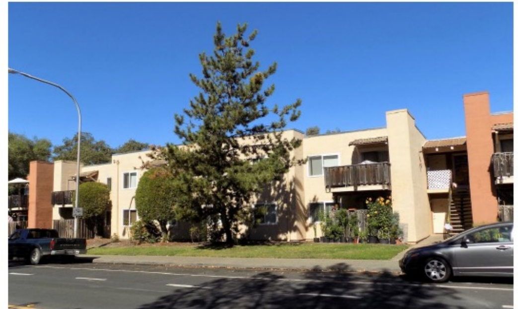
Monte Vina Apartments, pre-rehab
