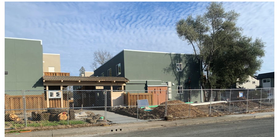
Monte Vina, nearing completion
